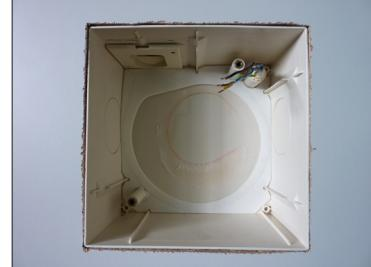
3. Place the seal, included in the scope of delivery, on the housing floor. When doing so, pay attention to the guide edges of the seal.
