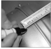
Mark the measure of C. Start from the joint of the fan.
