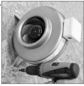
Mark the measure of **A** on the wall or roof and then fasten the fan.
