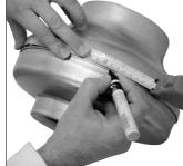
1. Mark the measure of B on the fan for the placement of the mounting brackets.
